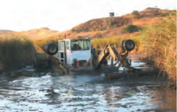
Silt must be cleared from channels so they can handle stormwater flows. In Fremont's Coyote Hills Regional Park, a device called an Aquamog floated in the waterway, clearing debris and vegetation with little impact to the natural setting.
