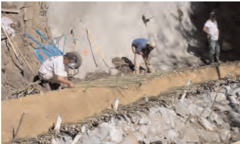
Each year, the District upgrades selected portions of its flood control infrastructure. Here, workers maximize the channel's capacity and stabilize its banks from erosion.
