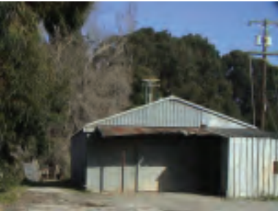
This spot alongside San Leandro Creek will be excavated to create an amphitheater with views of the restored creek stretch. The building shown will be renovated into an education center for visitors.
